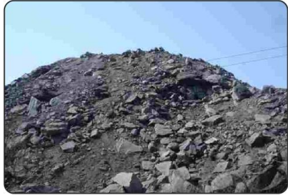
Over burden dump with 70° slope
