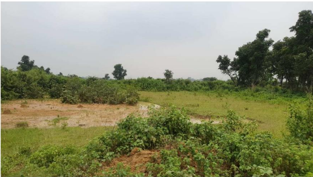
Figure 20: Subsidence (sag ponds) around Moonidih mine area
