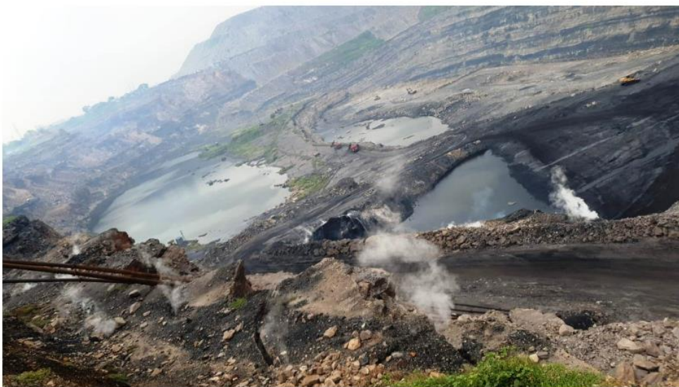
Figure 17: Fire in R-OCP. (Point 28 in figure 12)
