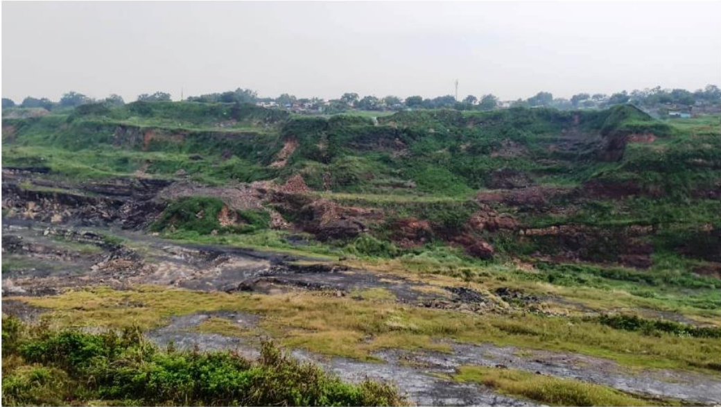
Figure 19: Subsidence area in Bagdigi Mines
